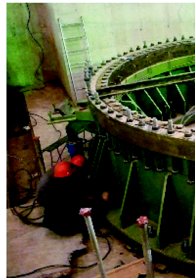
The On-site Installing of Anyang Steel Converter in Deyuquan Jiao
