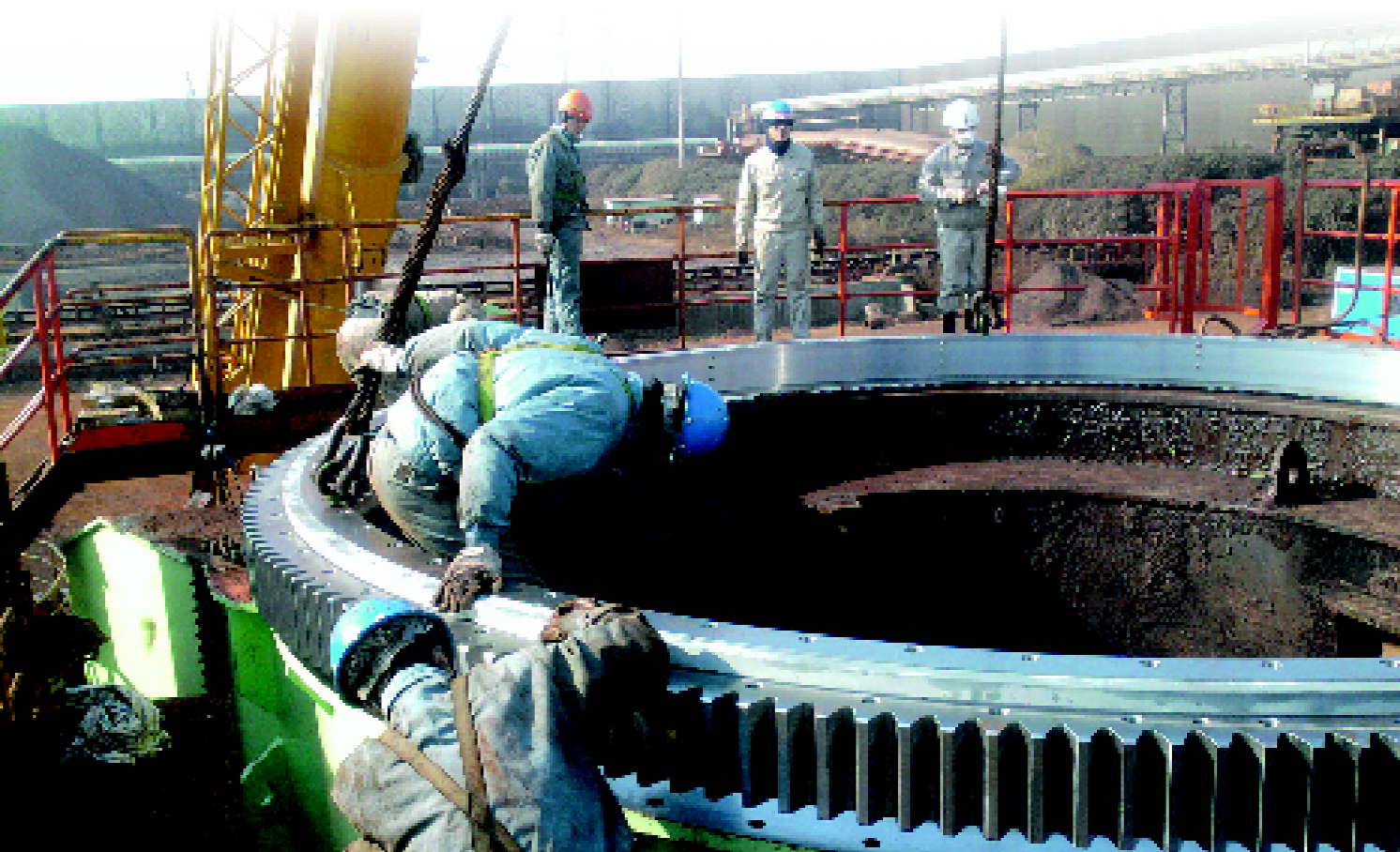
The On-site Installing of Baosteel 7500T Stacker-reclaimer
